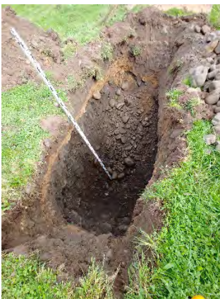
Left image: Site TP235 showing a sudden change in soil colour indicating there may have been disturbance at some point in time.
