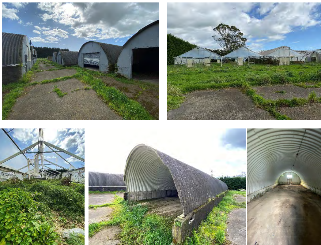
Figure 20 Out buildings located at 101 Waihou Road, Levin
